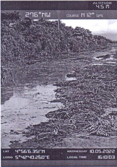
Fig B. SPILL POINT AFTER REPAIR
